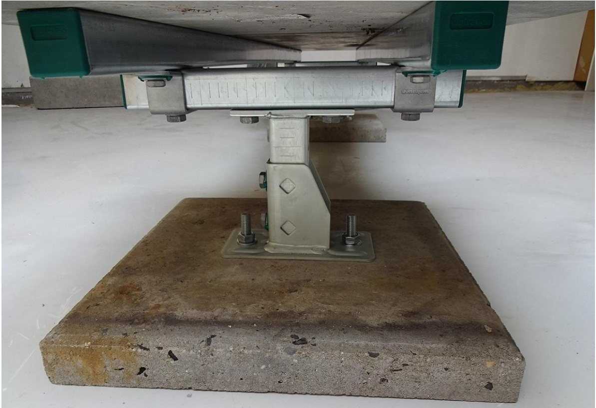
Photo 3: Reference construction, measurement 1, detail concrete slabs with rail base
