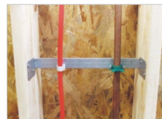
RSWB used in floor joists
