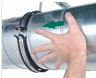
Trouble-free when sliding duct through clamp
