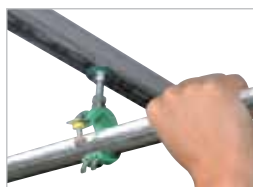
Place reinforced pipe into clamp
