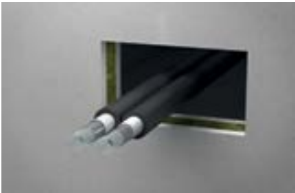
1. Clean the opening and check the dimensions
