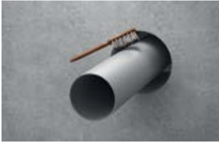
1. Clean the pipe and check the dimensions.
