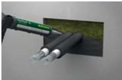
4. Apply the Walraven Pacifyre® G graphite fire sealant
