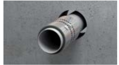
3. Bend and lock the tabs.
