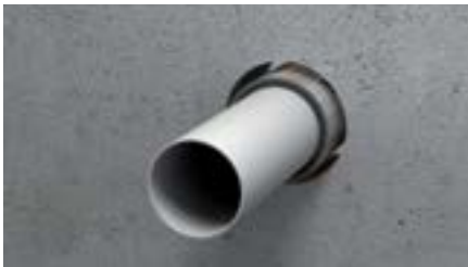
4. Slide the sleeve into the aperture and centre it.
