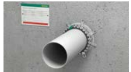
6. Fill out and place the Walraven Pacifyre® ID-Card next to the penetration.
