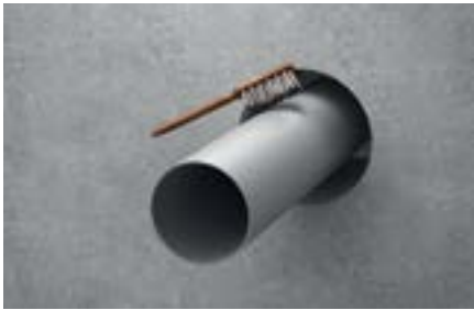
1. Clean the pipe and check the dimensions.
