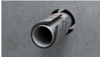
2. Fold the tabs in proper position.
