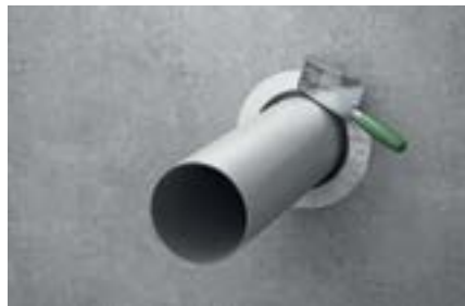
5. Flatten the acrylic with a jointing knife or trowel.
