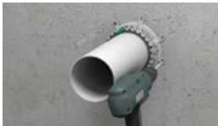
5. Mount the collar to the hole with an approved fixing set (as shown in the complementary products).
