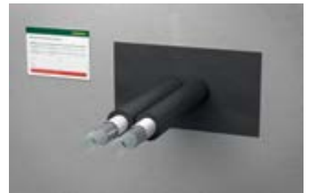
6. Place the filled out Walraven Pacifyre® ID-Card next to the penetration
