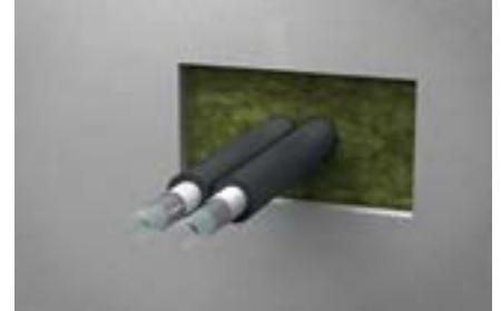
3. Check that the distance from the surface of the wall to the board is 25 mm
