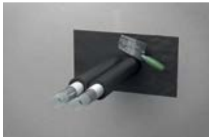
5. Flatten the Walraven Pacifyre® G graphite fire sealant with a jointing knife or trowel
