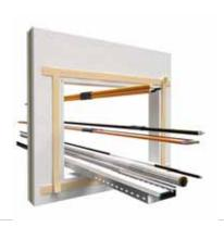
4. Cut the mineral fibre board to size (make cut-outs for the installations).
