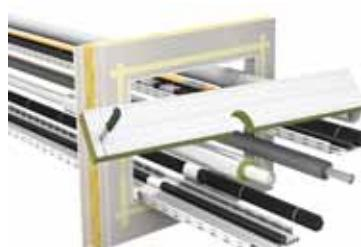
5. Coat the edges of the mineral fibre boards with Walraven Pacifyre® MWB-A and firmly place boards in position.
