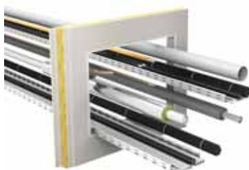
2. Mask the opening with crepe tape on all sides, keeping 20 mm distance to the edge. Coat the cables with Walraven Pacifyre® MWB-A; alternatively apply fire protection wrap.
