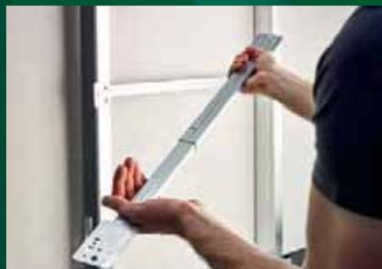
2. The brackets can be extended to fit between studs that are 16 to 24 inches apart.
