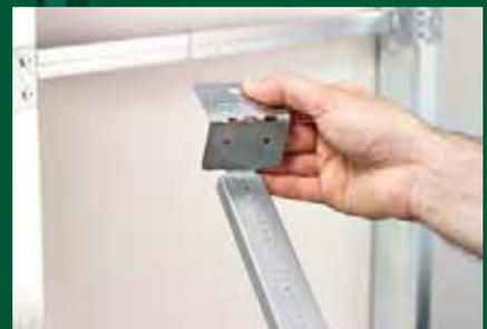
3. Bend the bracket ends to fix onto the studs.
