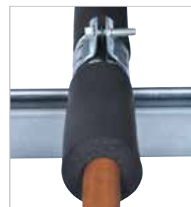
3. Place thermal insulation on pipe
