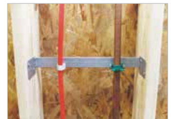
RSWB used in floor joists
