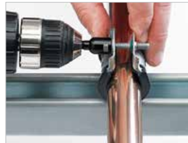
3. Tighten screw
