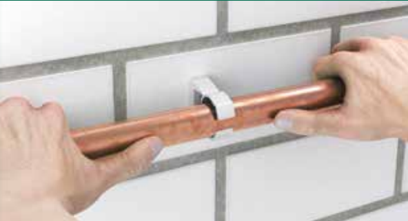
Push pipe into clamp.
