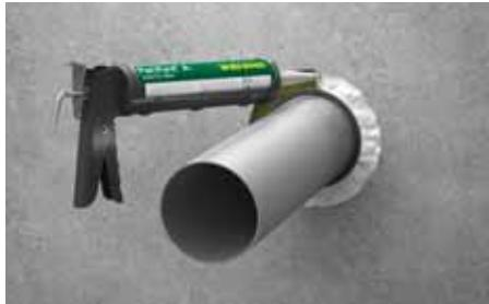
4. Seal the gap with Pacifyre® A Acrylic Sealant ( $t = 10$  mm).
