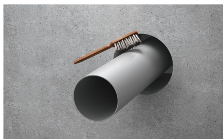
1. Clean the pipe and check the dimensions.
