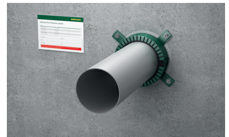
6. Fill out and place the Walraven Pacifyre® ID Card next to the penetration.
