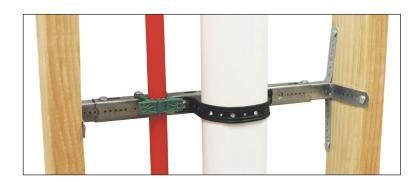
MPTS used with suspension band to hold drain pipe and Rabbit clamp to hold PEX.
