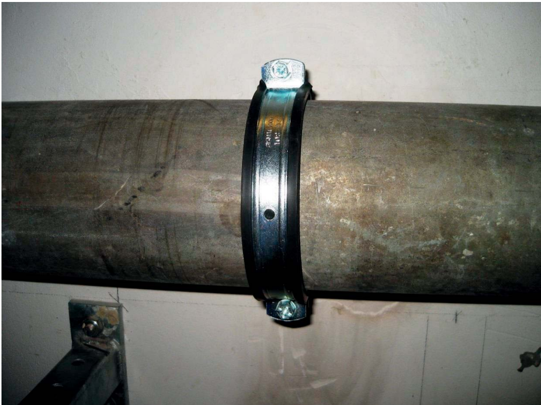
Fig. 2: Meas. 4: BISMAT® 2000, 4" (108 - 114mm), connection M8/10, with EPDM-rubber (25 x 4,00 mm)
