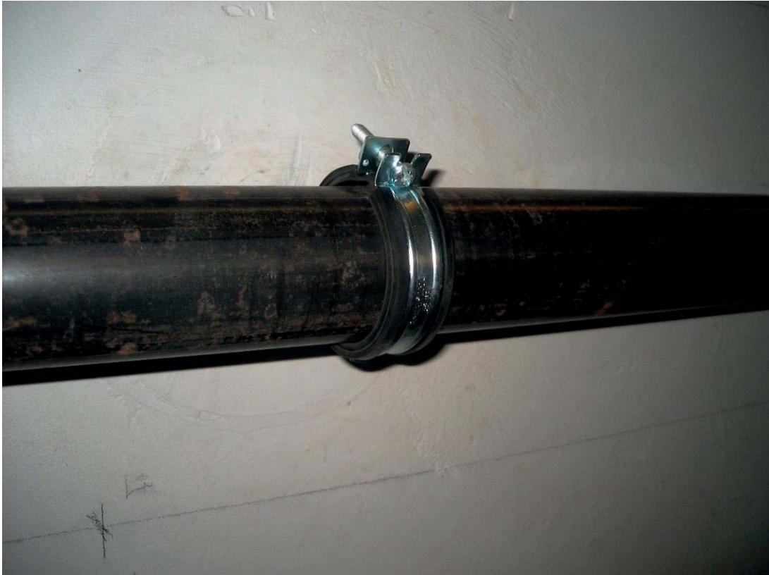
Fig. 1: Meas. 3: BISMAT® 2000, 2" (58 - 63mm), connection M8/10, with EPDM-rubber (20 x 4,20 mm)
