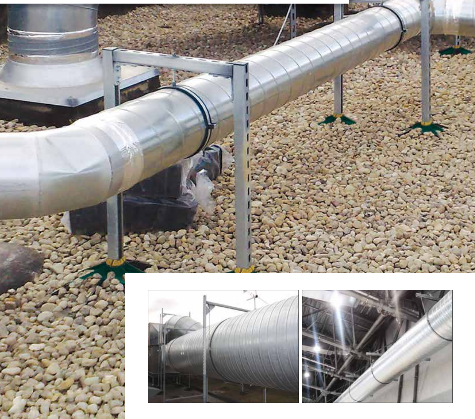
Rubber lining is conjoined with the clamp
