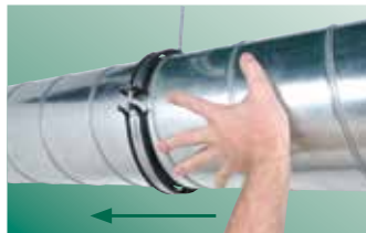
Trouble-free sliding of spiral duct clamp
