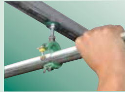
Place reinforced pipe into clamp
