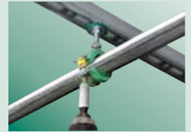
Final tighten assembled clamp
