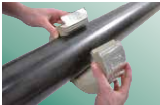
1. Ensure correct size of block. Lift sealing tag, open block and position around pipe.
