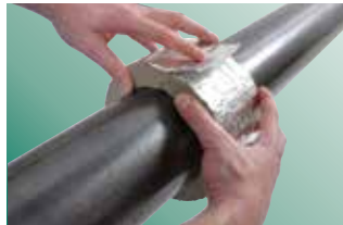
2. Close block around pipe and re-seal tag.
