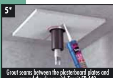
Grout seams between the plasterboard plates and around the sleeve with Tangit FP 440
