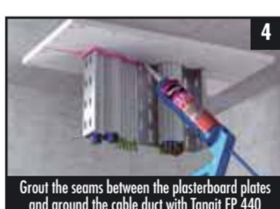
Grout the seams between the plasterboard plates and around the cable duct with Tangit FP 440
