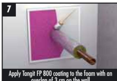
Apply Tangit FP 800 coating to the foam with an overlap of 3 cm on the wall
