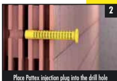
2 Place Pattex injection plug into the drill hole
