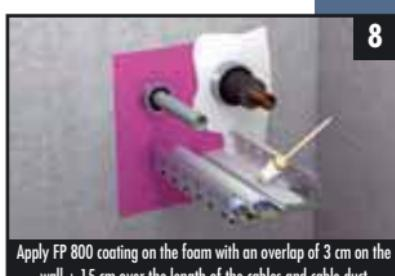
Apply FP 800 coating on the foam with an overlap of 3 cm on the wall + 15 cm over the length of the cables and cable duct
