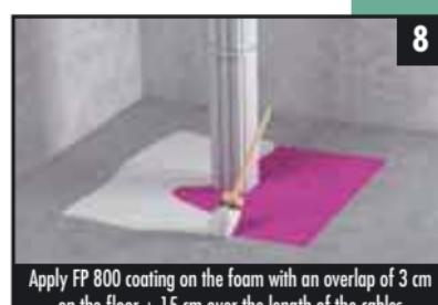
Apply FP 800 coating on the foam with an overlap of 3 cm on the floor + 15 cm over the length of the cables
