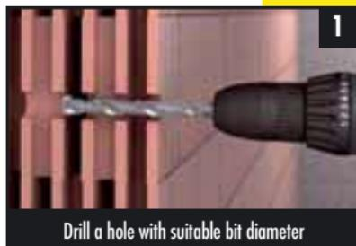
1 Drill a hole with suitable bit diameter
