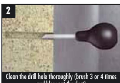
2 Clean the drill hole thoroughly (brush 3 or 4 times and blow out the dust)
