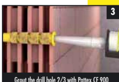
3 Grout the drill hole 2/3 with Pattex CF 900
