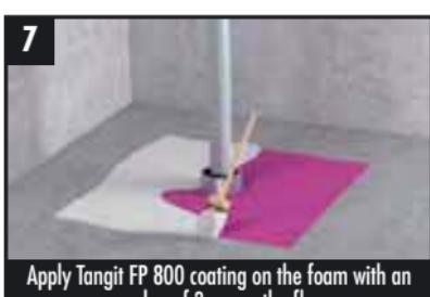
Apply Tangit FP 800 coating on the foam with an overlap of 3 cm on the floor
