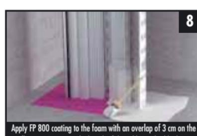
Apply FP 800 coating to the foam with an overlap of 3 cm on the floor + 15 cm over the length of the cables and cable duct
