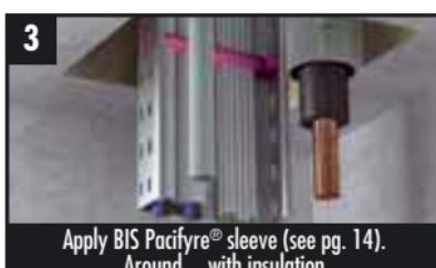
Apply BIS Pacifyre® sleeve (see pg. 14). Around...with insulation
