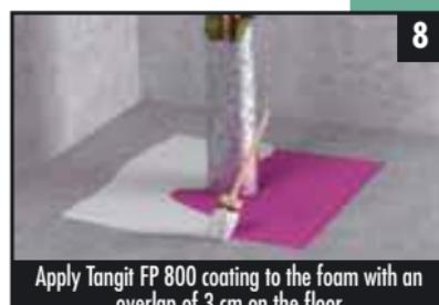
8 Apply Tangit FP 800 coating to the foam with an overlap of 3 cm on the floor
