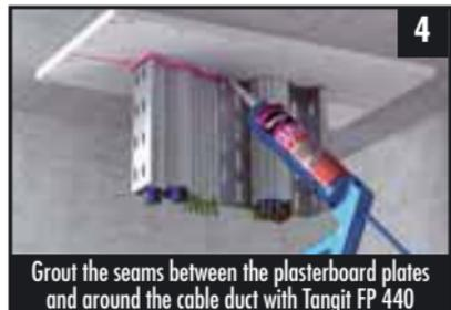
4 Grout the seams between the plasterboard plates and around the cable duct with Tangit FP 440
