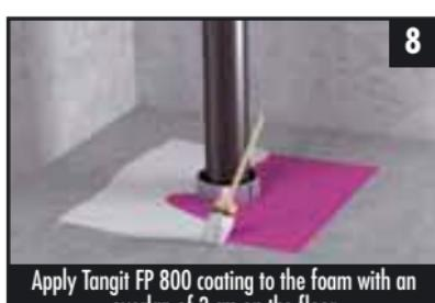
Apply Tangit FP 800 coating to the foam with an overlap of 3 cm on the floor
