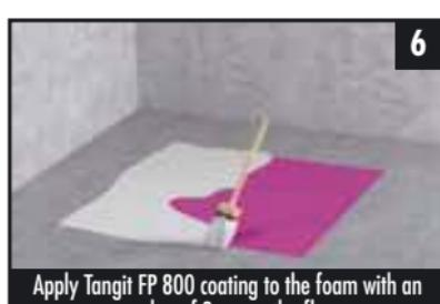
6 Apply Tangit FP 800 coating to the foam with an overlap of 3 cm on the floor
