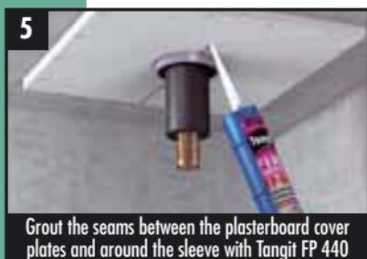
Grout the seams between the plasterboard cover plates and around the sleeve with Tangit FP 440
