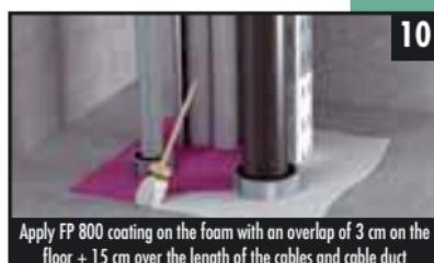
Apply FP 800 coating on the foam with an overlap of 3 cm on the floor + 15 cm over the length of the cables and cable duct
