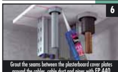
Grout the seams between the plasterboard cover plates around the cables, cable ducts and pipes with FP 440
