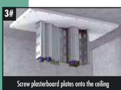
Screw plasterboard plates onto the ceiling
