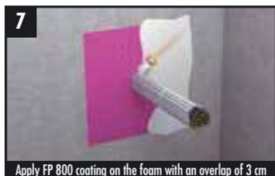
Apply FP 800 coating on the foam with an overlap of 3 cm on the wall + 15 cm over the length of the cables
