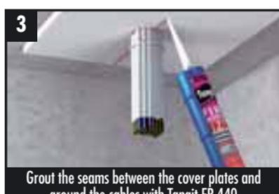
Grout the seams between the cover plates and around the cables with Tangit FP 440
