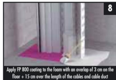
8 Apply FP 800 coating to the foam with an overlap of 3 cm on the floor + 15 cm over the length of the cables and cable duct
