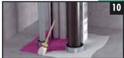
10 Apply FP 800 coating on the foam with an overlap of 3 cm on the
