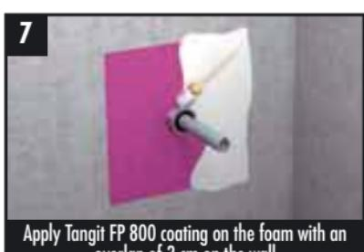
7 Apply Tangit FP 800 coating on the foam with an overlap of 3 cm on the wall
