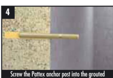
4 Screw the Pattex anchor post into the grouted drill hole (counter clockwise)
