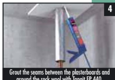
4 Grout the seams between the plasterboards and around the rock wool with Tangit FP 440.
