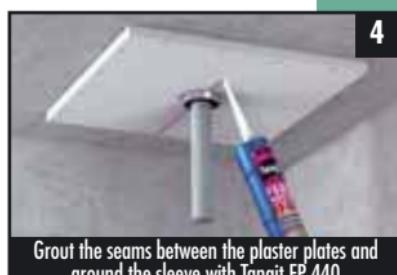
Grout the seams between the plaster plates and around the sleeve with Tangit FP 440
