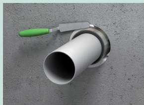
5. Fill the opening with Fire resistant acrylic or mortar
