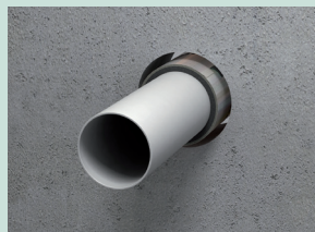
4. Slide the sleeve into the aperture and center it
