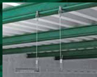
For cable trays
