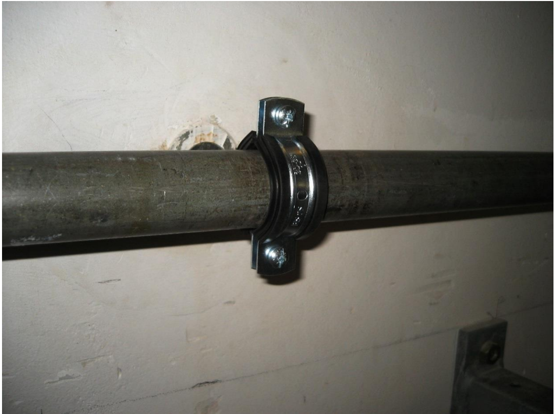
Fig. 1: Meas. 2: BIS Schelle 2S, 1" (30 - 35mm), connection M8/10, with EPDM-rubber (20 x 3,70 mm)
