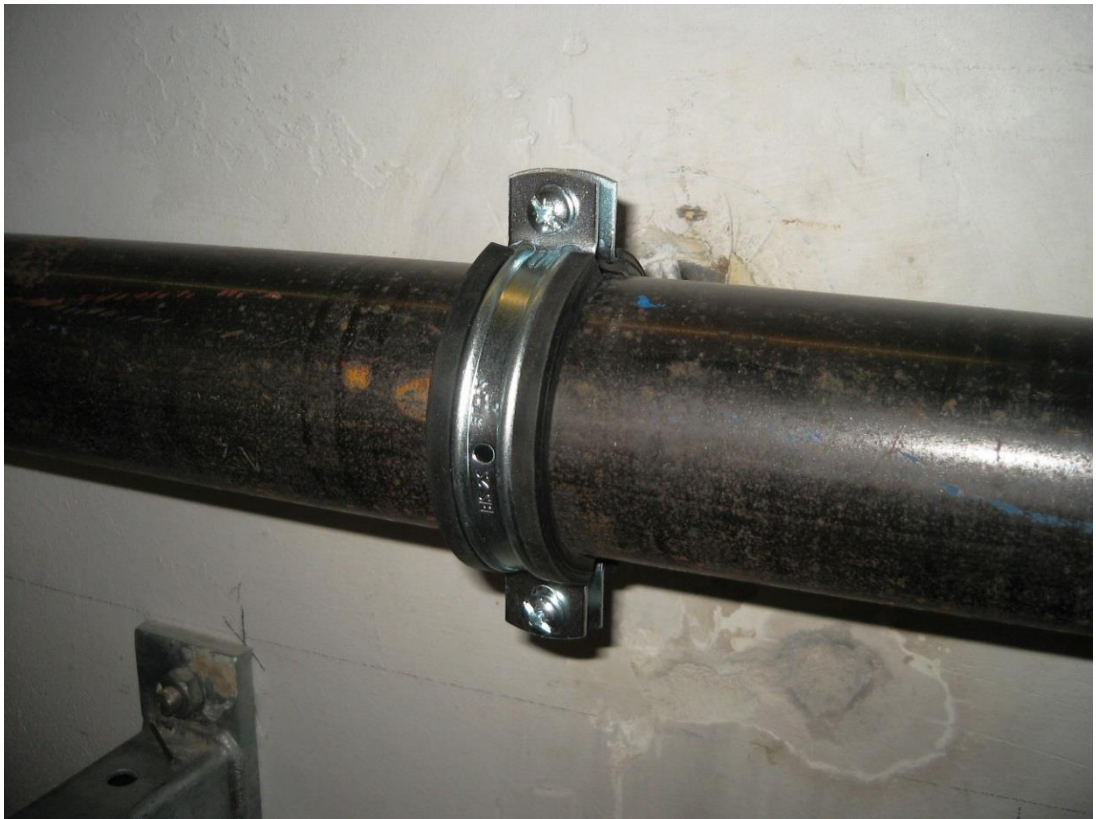
Fig. 2: Meas. 3: BIS Schelle 2S, 2" (57 - 63mm), connection M8/10, with EPDM-rubber (20 x 4,00 mm)
