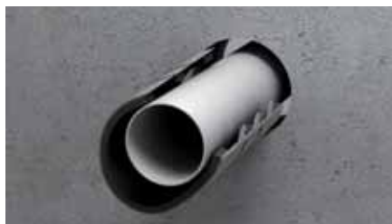
1. Wrap the sleeve around the pipe
