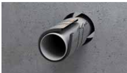
2. Fold the tabs in proper position
